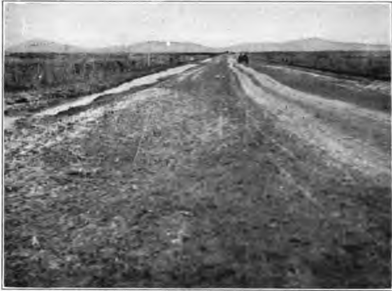
FIG. 7. OLD ROAD IN SANPETE COUNTY SHOWING RESULTS OF CONSTRUCTING A WIDE ROAD.
